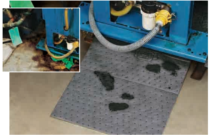
Machine Leaks and Drips
